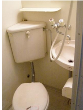
Fixed Type Bathroom (Building A & B)
