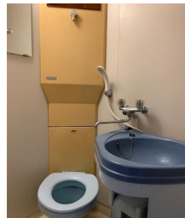
Rotary Type Bathroom (Building C, D, E, F)
